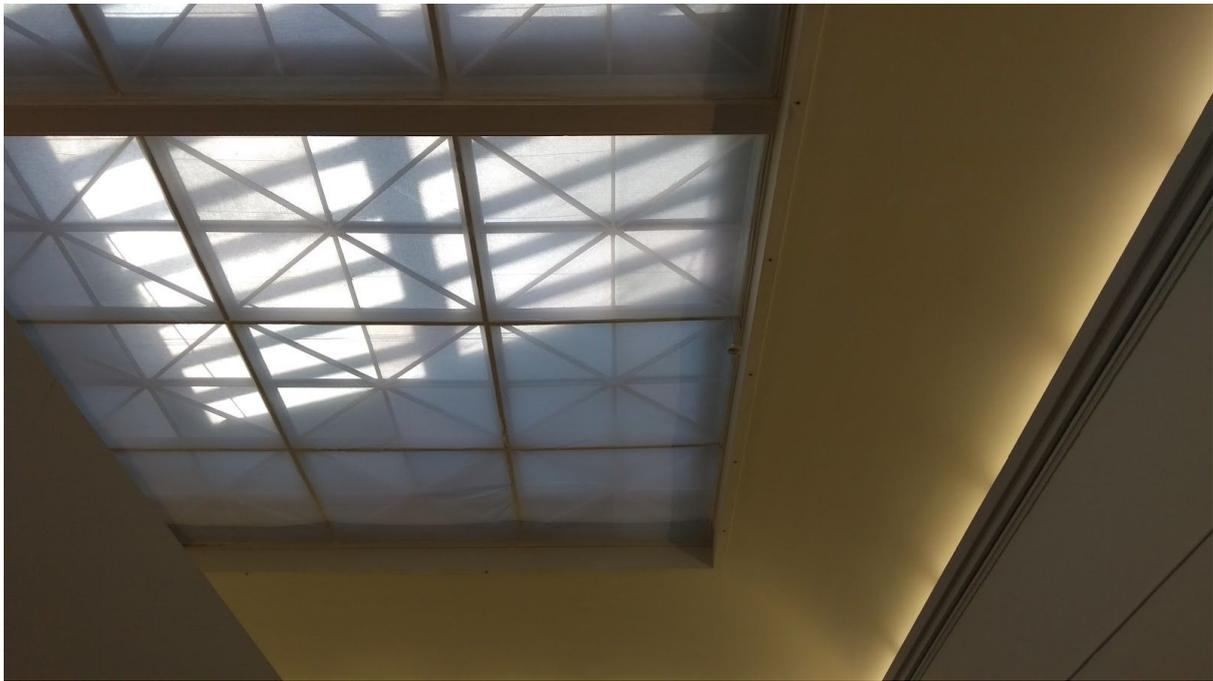
Image shows: safety net installed in the ceiling of Gothenburg Konsthall, a prerequisite for showing the work. Photo: Karl Bergström, 2017.
